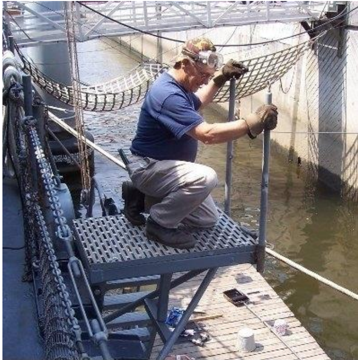
"Super" Dave Mardon rigging the safety railing on the accommodation ladder.
