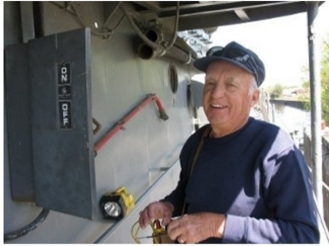
Larry Williams disconnects the shore tie on move day.
