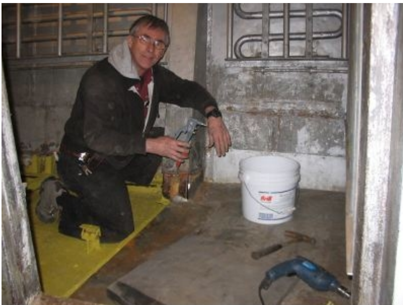
Gary Sheedy replacing the false decking in the starboard reefer.
