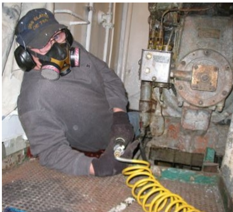
Gary Lubrano scaling the high pressure air compressor in B-3.
