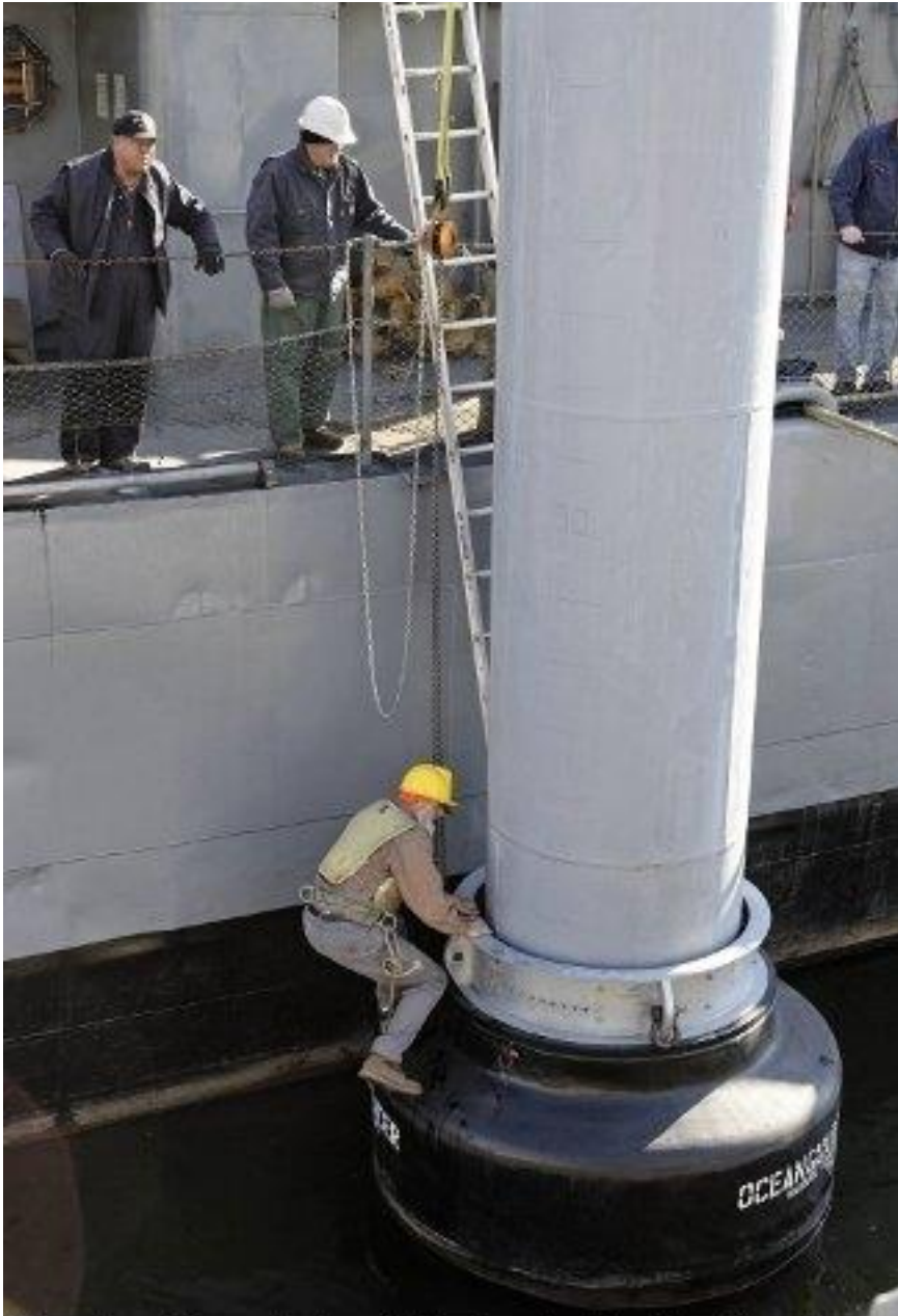
Rigging the chain falls to hoist the fenders.
