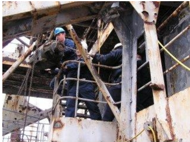
Rigging out a motor generator set for removal from the GAGE.
