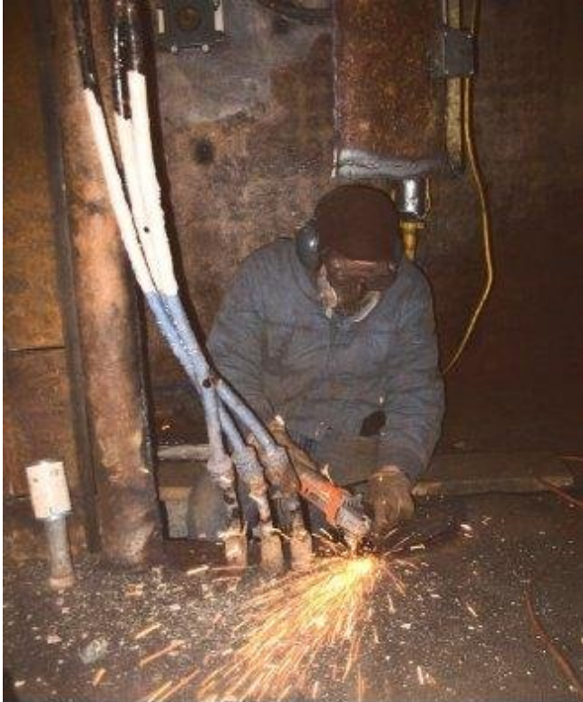
Gene Jackey grinds off the remains of a tripled bulkhead.
