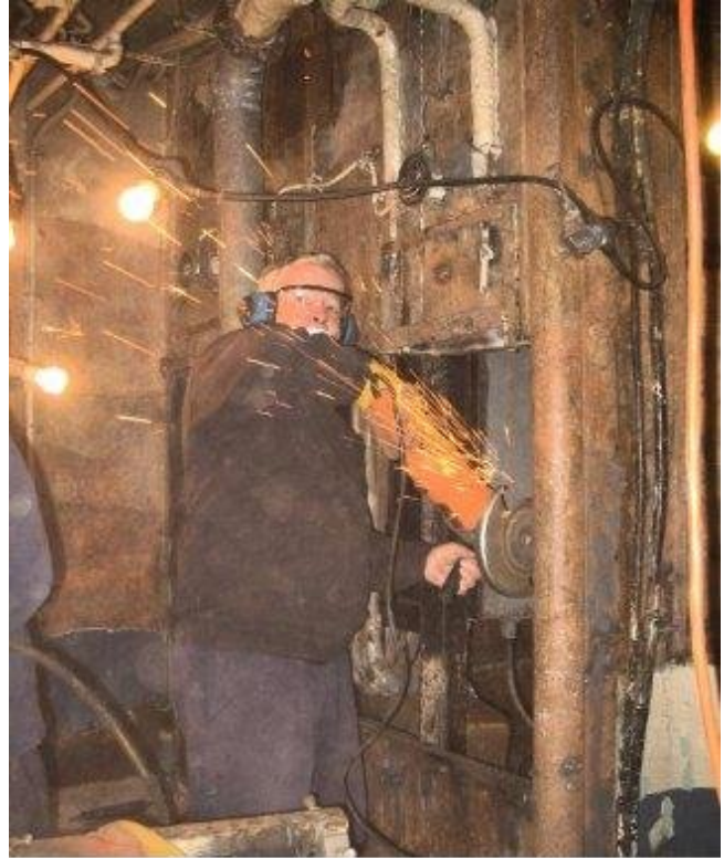
At the other end of the compartment Earl Herchenroder grinds a bulkhead.
