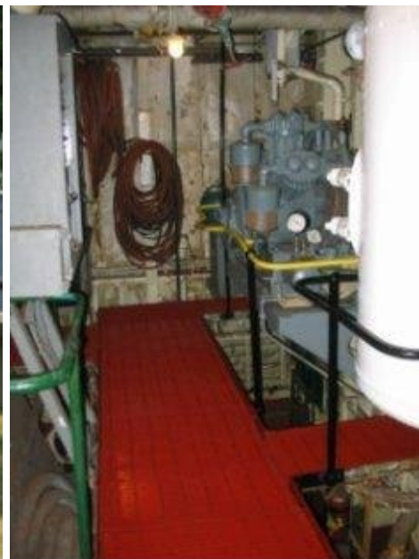
Repainted B4 deck plates, air tank and compressor.
