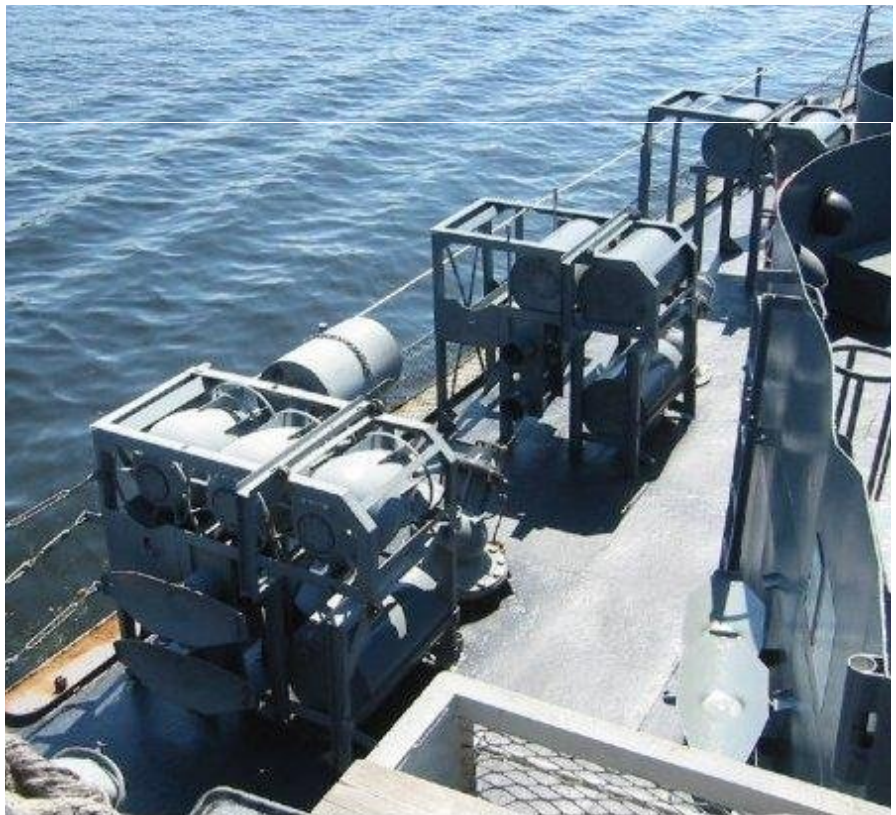
An original depth charge rack in the foreground with two partially complete racks in the background.
