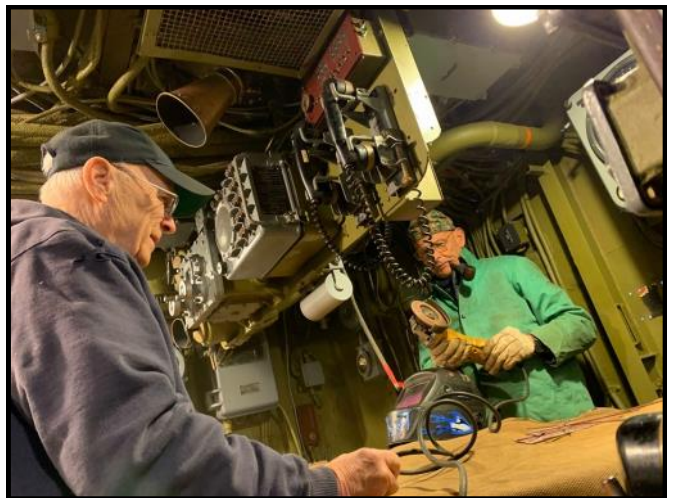
This can't be good. Shipfitters Dave Mardon and Tim Benner working in CIC.
