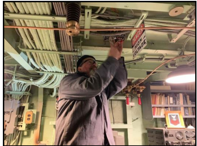
Steve Klauck installing a smoke detector in the radio shack
