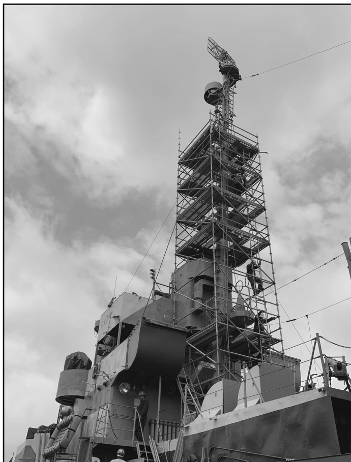
Day 3 in the shipyard. Yardarm is removed and scaffolding is up.
