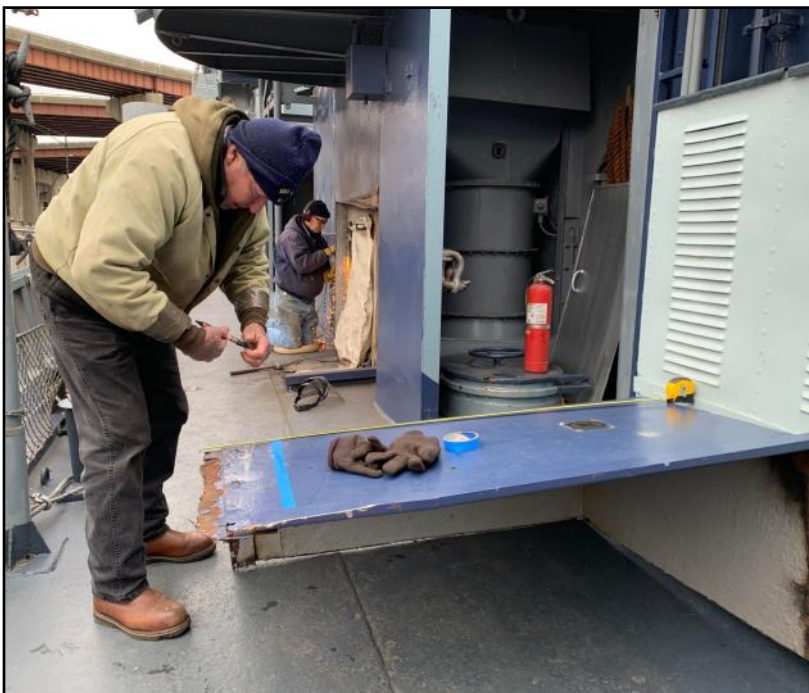
Danny and the shipfitters continue to work on the supply vent.
