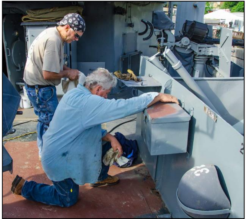
Rick Espenshade and Steve Wulko patching holes in the deck.
