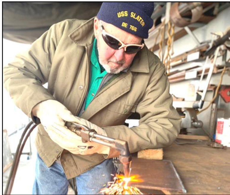
Danny cutting a plate to patch the signal bridge.
