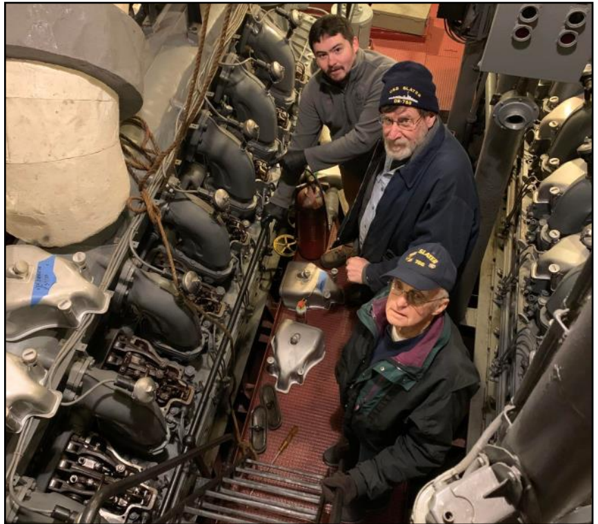
James, Jim, and Larry continue to work on diesel restoration and bilge preservation.
