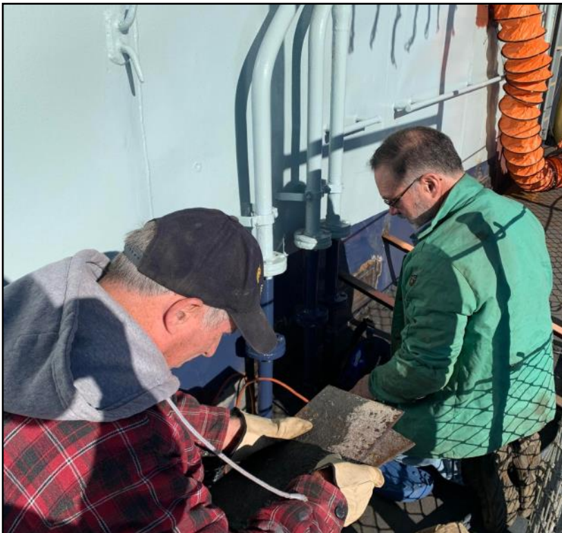
Bill has just about completed the welding in the wardroom.
